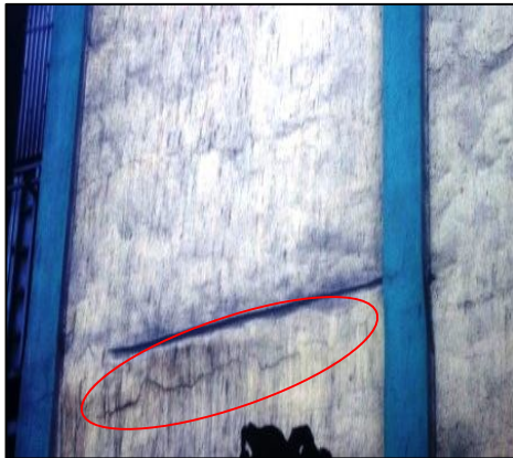
Horizontal cracks with undulation
