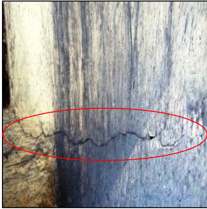
Horizontal cracks and seepage mark noted.
