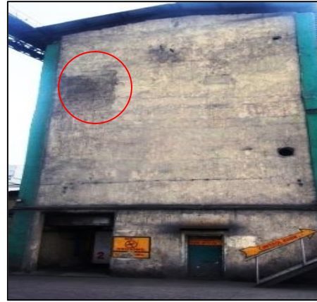
Horizontal cracks and seepage mark noted.
