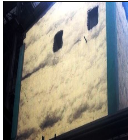
Undulation and cracks noted at external facade.
